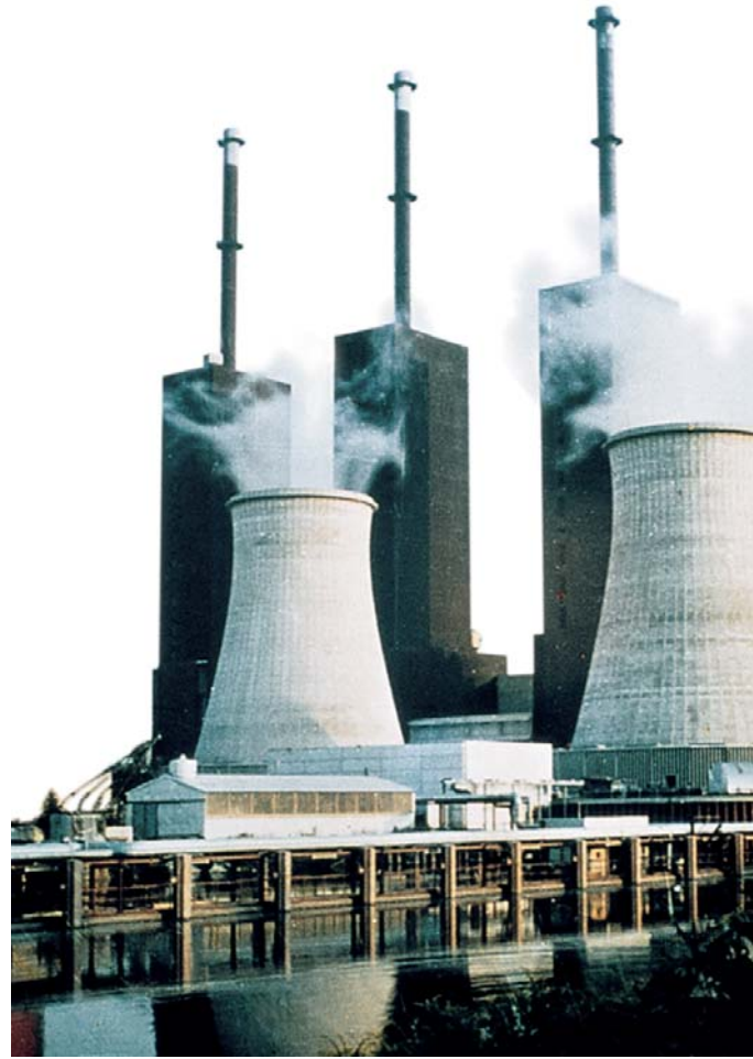
Circular cooling towers with forced draught fans at a combined heat and power station
