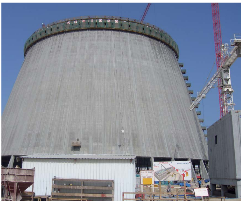
Circular cooling tower under construction
