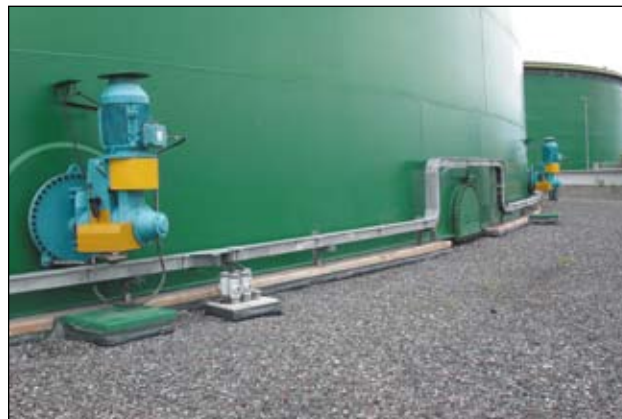
Plenty swivel angle gear drive mixer complete with automatic actuator
