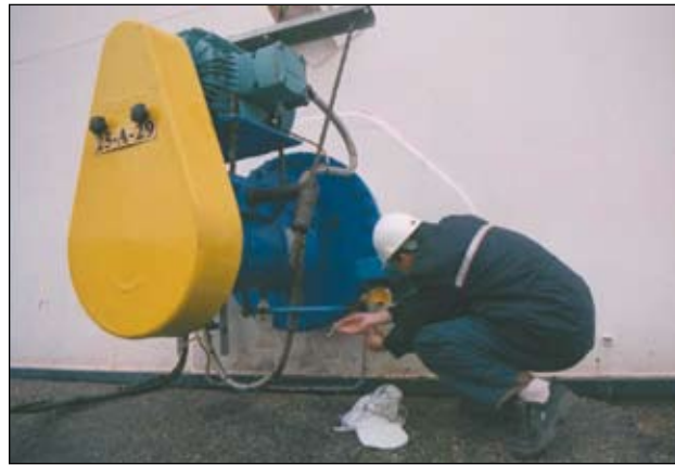
Final installation of a Plenty belt drive mixer
