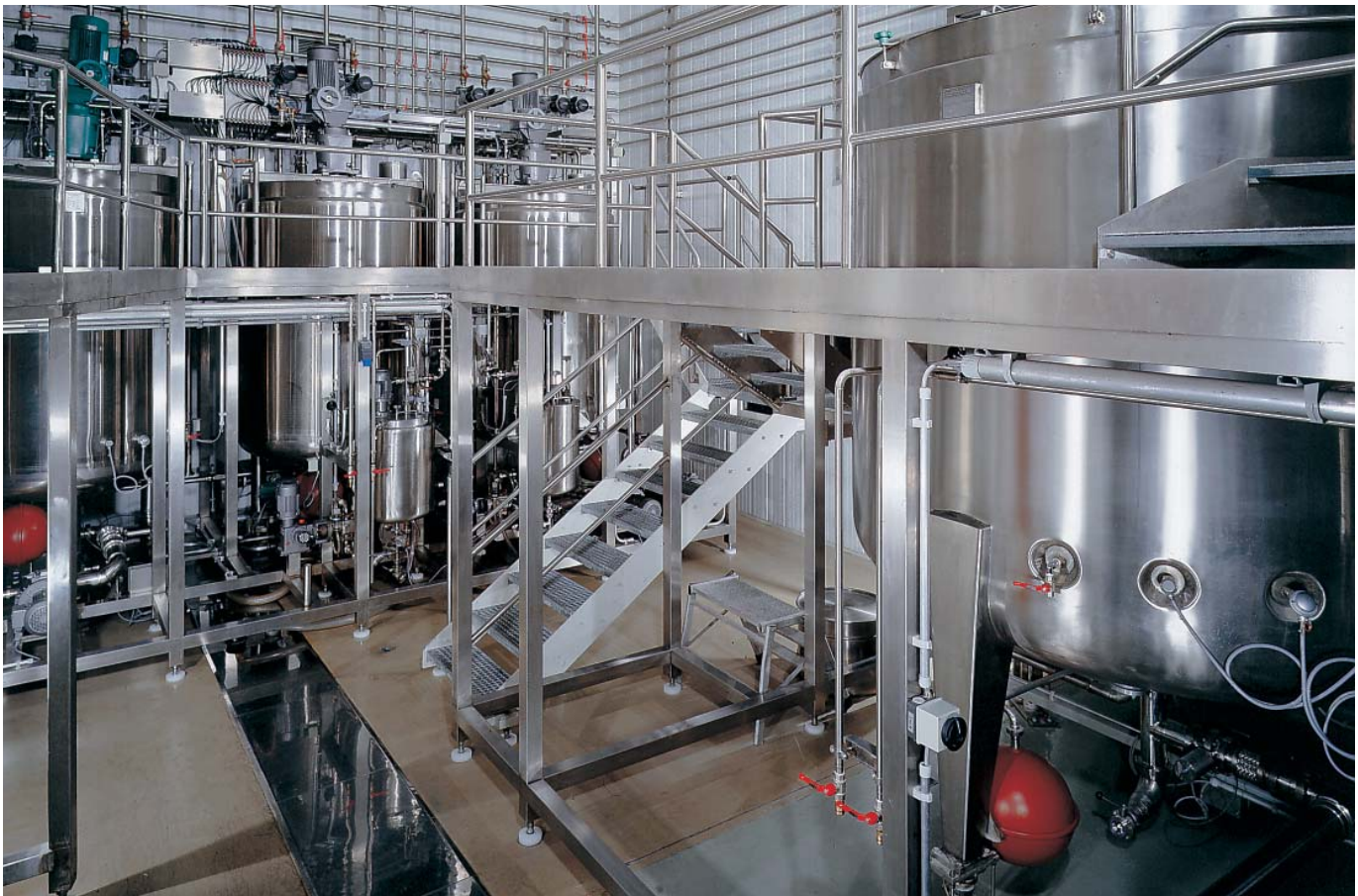
Production of lotion and detergent in parallel batch containers. Gravimetric control for primary components. Minor components are metered in from separate containers.
