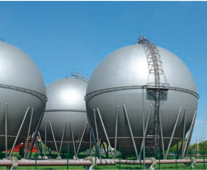
Odourizing of natural gas
