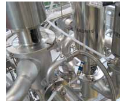
CIP run-off for sampling valves protects fittings and pumps (left)
