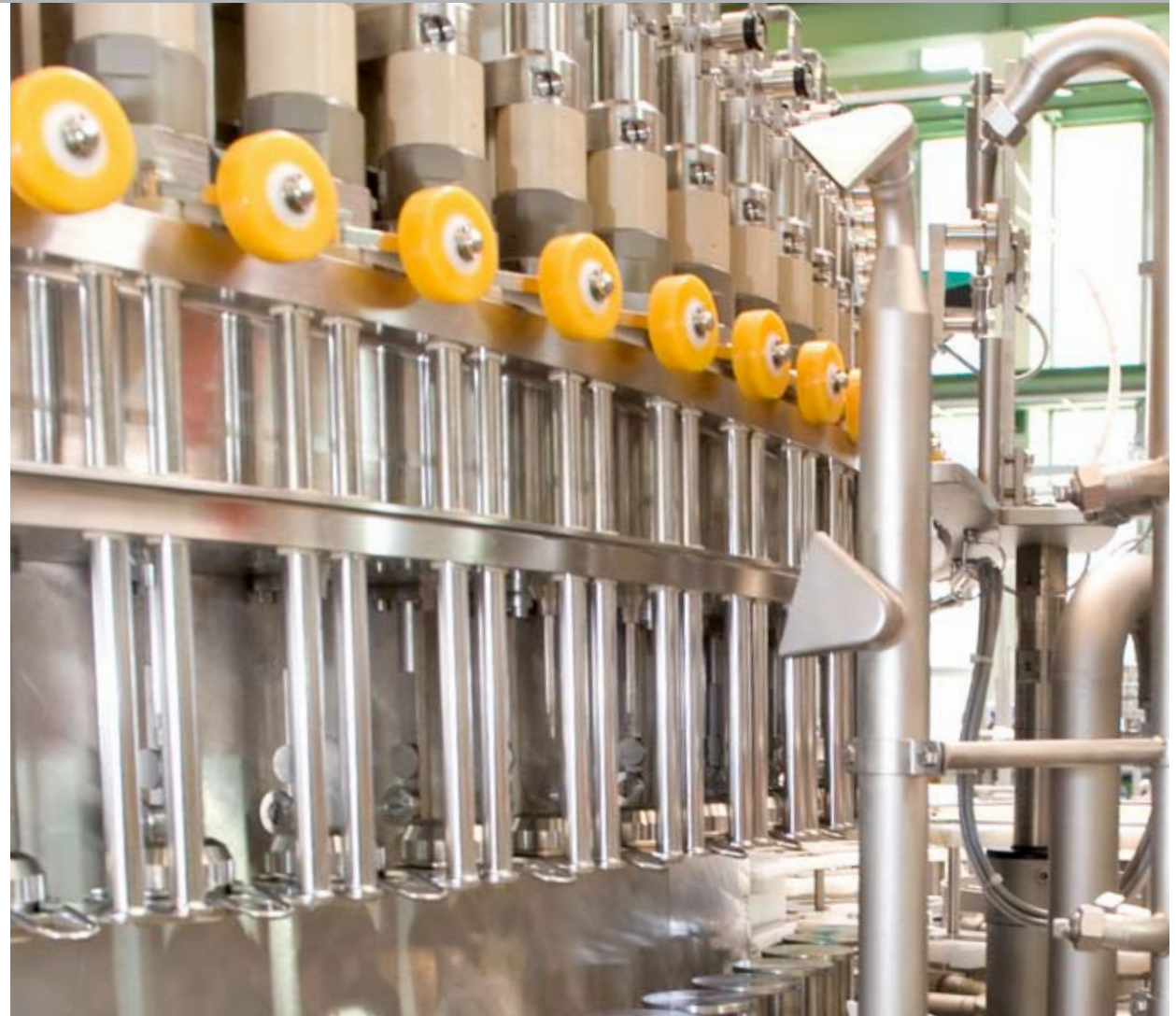
Flushing system for cleaning the outside
