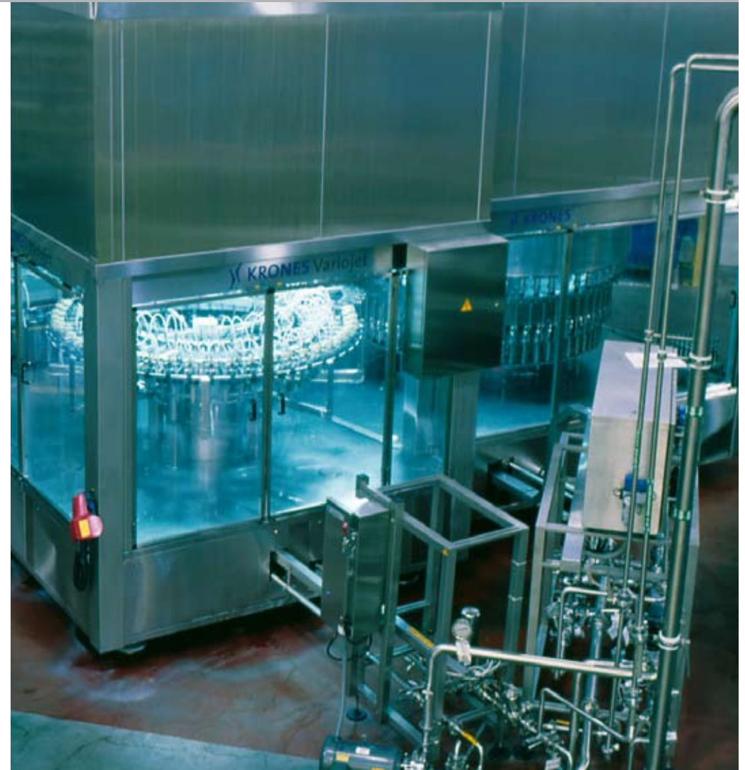
Clean room housing
