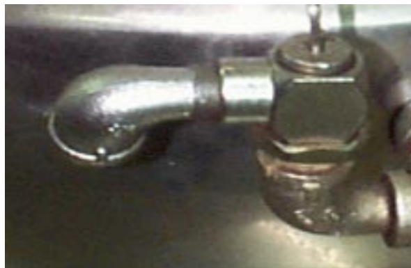
The open end of the pop safety valve elbow must face downward.
