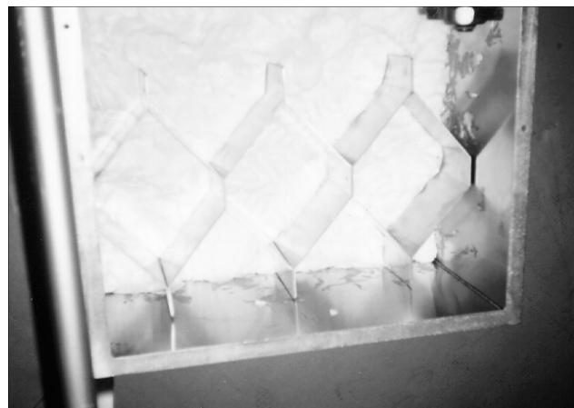
Figure 1-8. Installing the Cube Melter.
